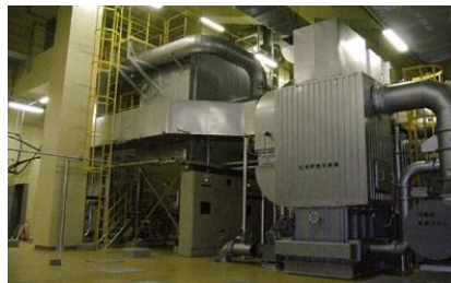
Figure 7: Japanese cremation system with modern emission treatment equipment
